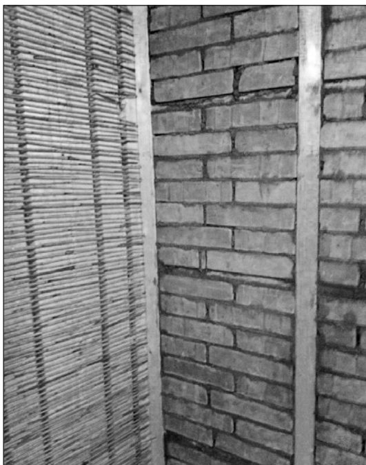
Figure 6: Accumulation wall of mud bricks – House, Slovakia
