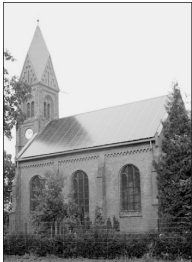
Figure 2: Example of roofing materials, using solar energy and at the same time are so made that at first glance do not differ from shale or from metal sheet - church in Wieck, Germany
