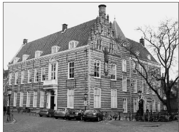
Figure 7: The Pope's House, Utrecht, the Netherlands
