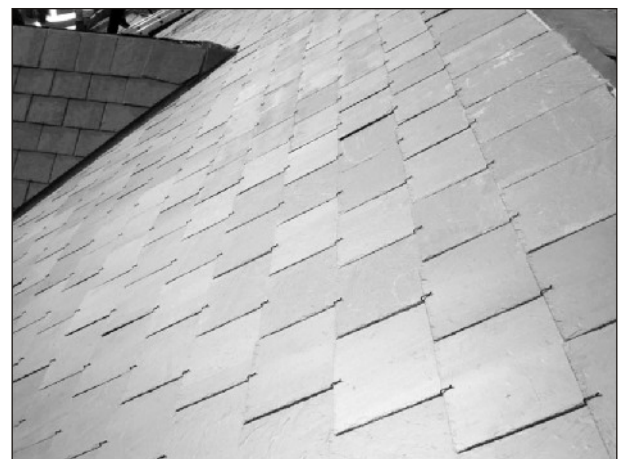
Figure 4: Solar tiles on the roof of a traditional building used primarily on the British Isles.
